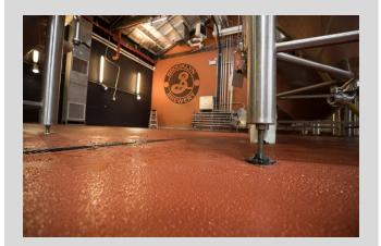
Flowfresh material is highly durable offering excellent thermal cycling and thermal shock resistance. This makes the material ideal for installation in areas subject to extremely hot temperatures or those that may be exposed to intermittent hot spillage or hot water wash down processes.
